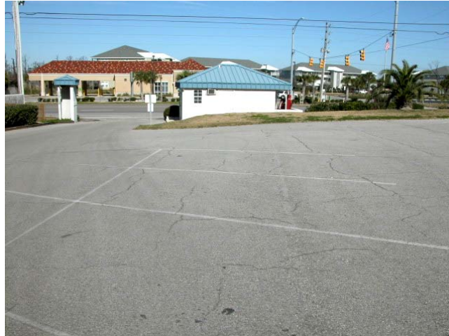
Asphalt paving in parking area.
