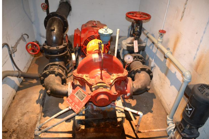
Fire pump and its accessories were found to be in good condition
