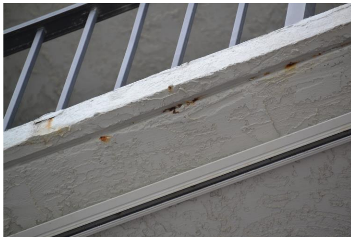
Rust spots forming on the concrete of a balcony.
